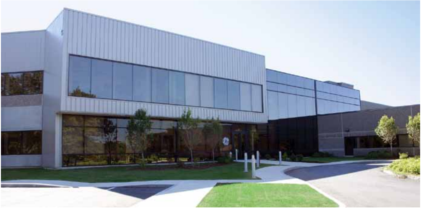
GE Measurement & Control Solutions building in Billerica, Massachusetts, USA
